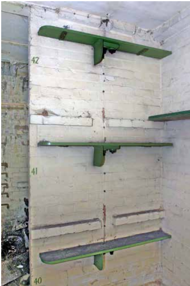
One of the numbered sleeping bays with a shelf and a light provided for each of the three bunks
